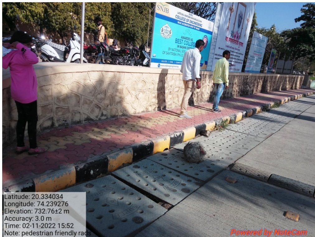
Figure 3. Well constructed Foot paths on main Road in the campus
