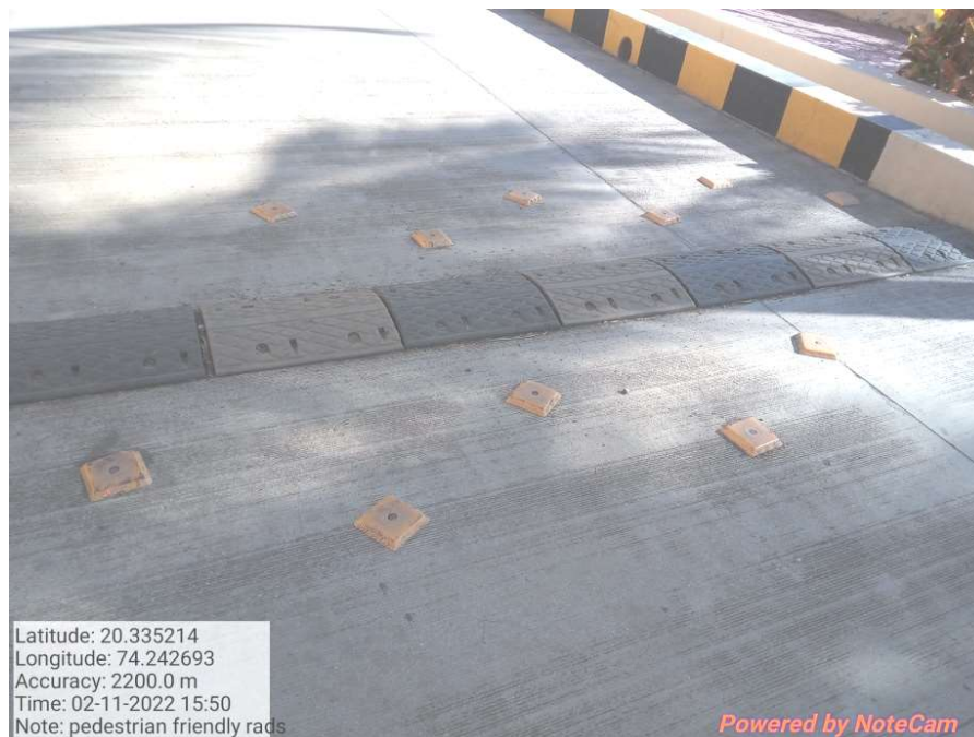
Figure 1 Speed breakers at the divergent roads
